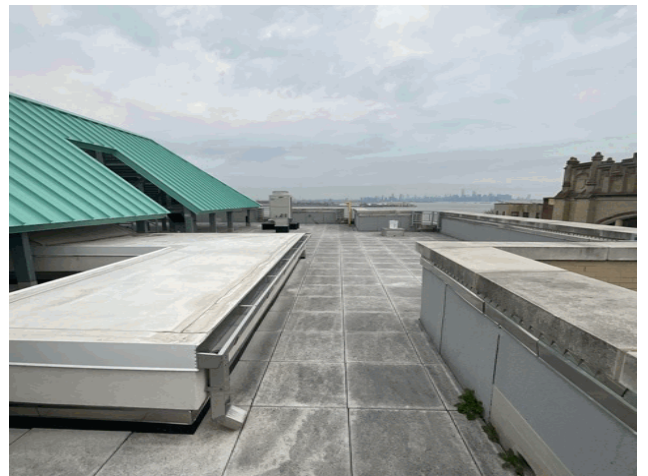
Roof 1 - North View
