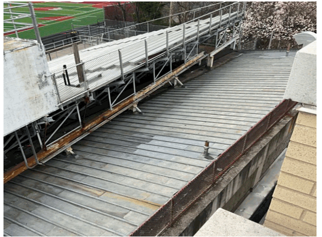
Roof 1 - Southwest View
