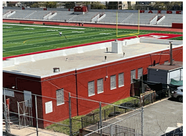
Roof 1 - North View from Main Asset R445
