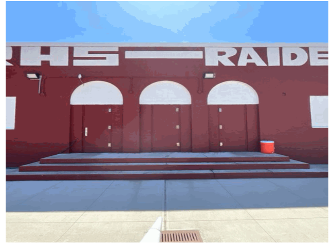
Facade A - From Football Field
