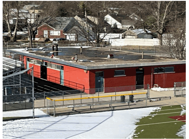
Roof 1 - West View
