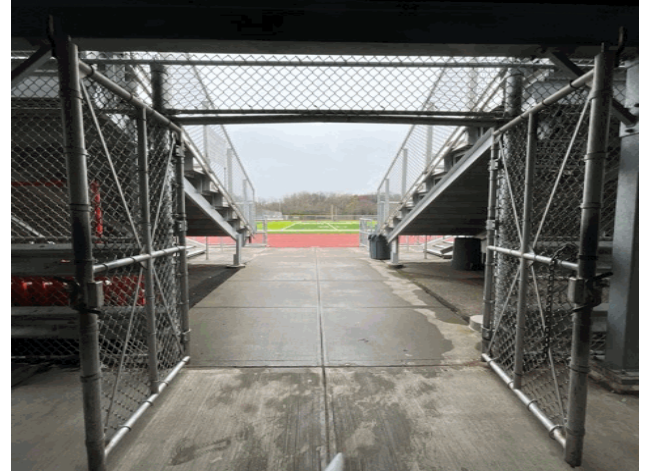
Main Entrance Gate
