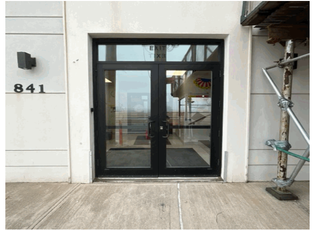
Facade A - Father Capodanno Boulevard
