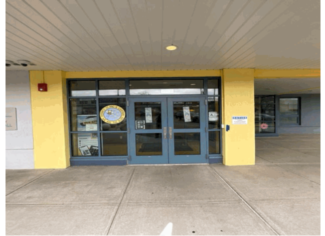
Facade A - Lynhurst Avenue
