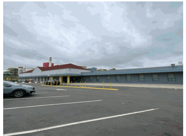
Lynhurst Avenue - West View
