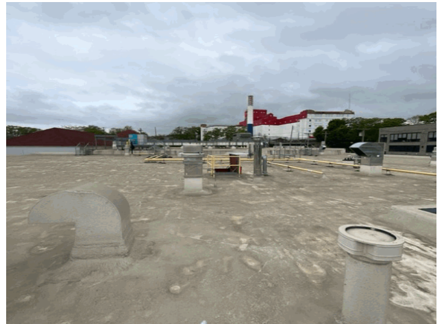
Roof 1 - West View
