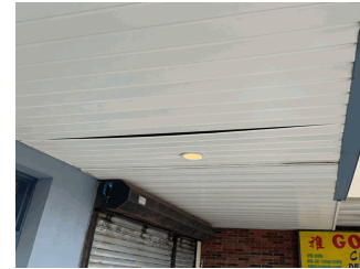
Facade A - Right of Exit 3
