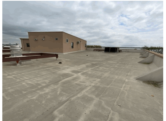
Roof 1 - Northeast View
