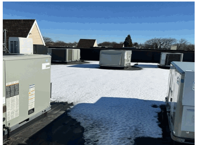
Roof 1 - Northeast View
