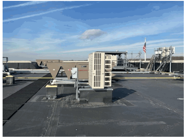
Roof 1 - Northwest View
