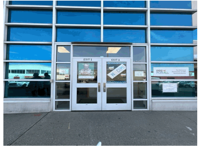
Facade A - Richmond Avenue Parking Area
