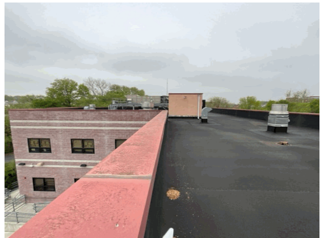
Roof 1 - South View
