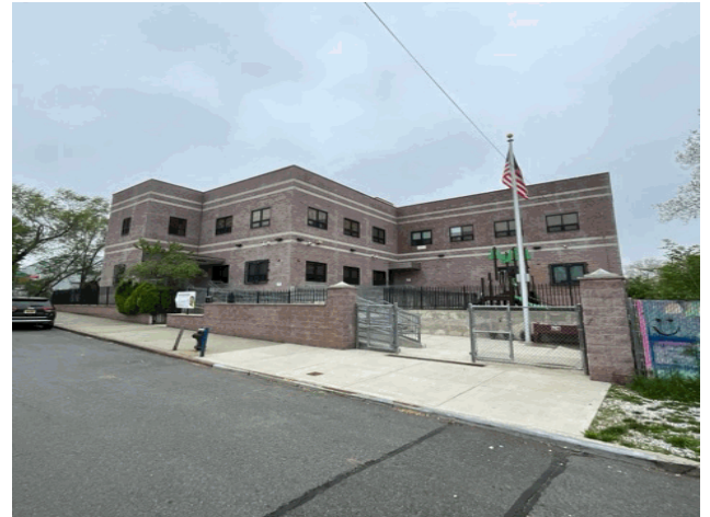
Housman Avenue - Southwest View
