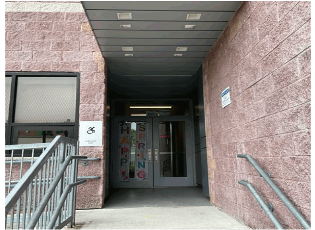
Facade A - Housman Avenue
