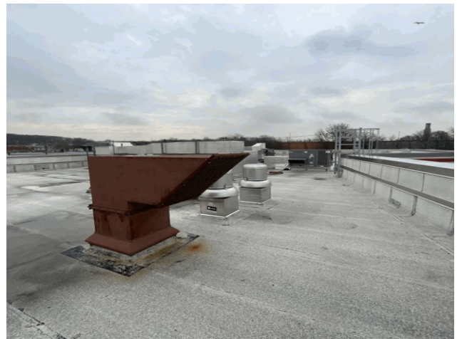
Roof 1 - South View
