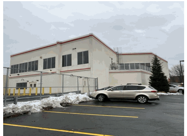
Corner of Wyona Place and Victory Boulevard - South View
