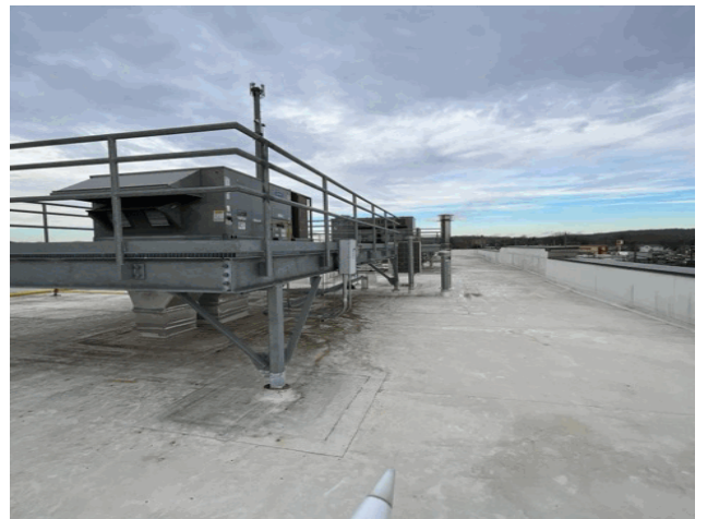
Roof 1 - West View
