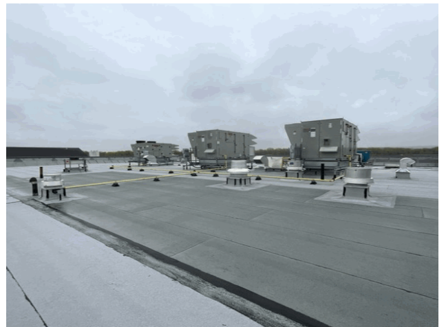
Roof 1 - North View
