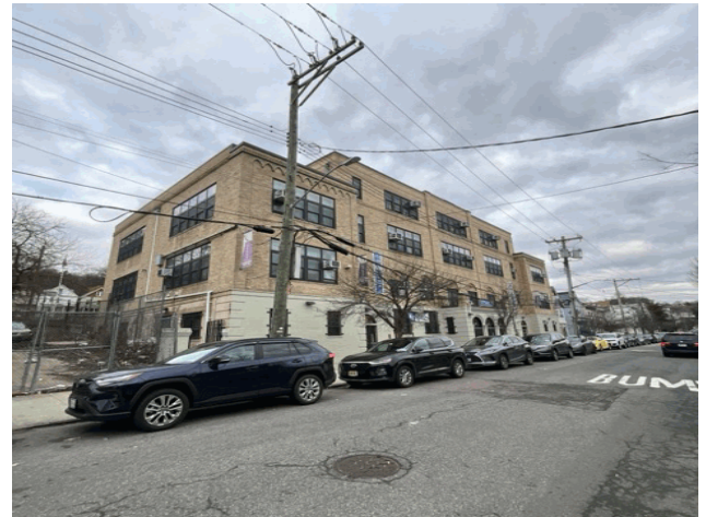
Gordon Street - North View
