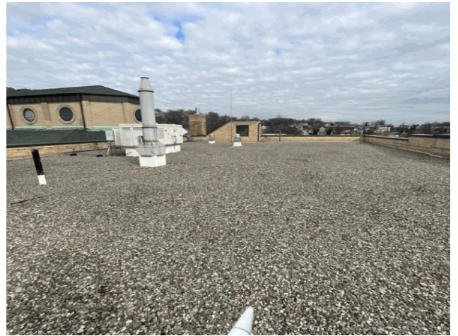
Roof 1 - North View
