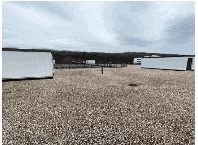
Roof 1 - South View
