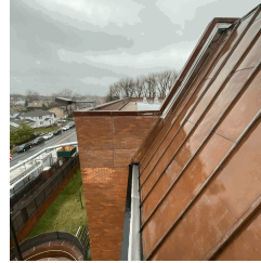
Roof at Bulkhead A
