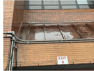
Roof at Exit 8 Vestibule
