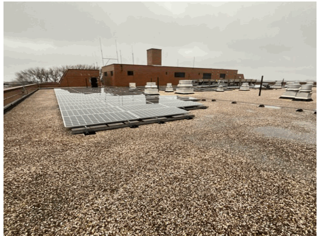
Roof 1 - North View
