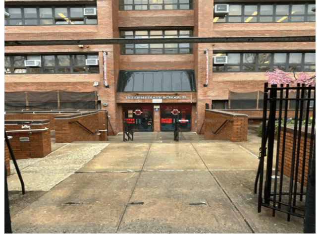
Facade A - Huguenot Avenue
