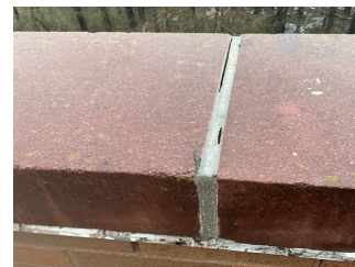
Roof 1 - Facade G
