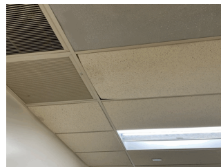
Corridor near Room 405 shown, also Rooms 106 and 405 No photo recorded
