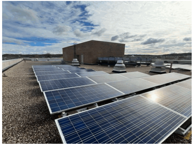
Roof 1 - East View
