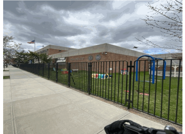
Keating Place - West View
