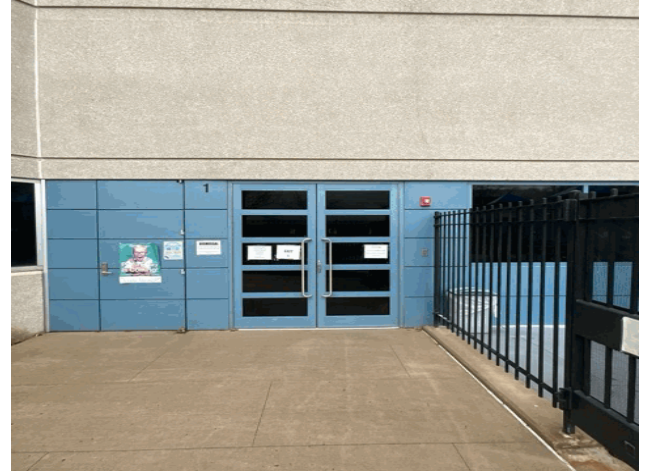
Facade A - Teleport Drive
