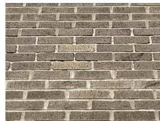
Facade C over Room 114 Exit
