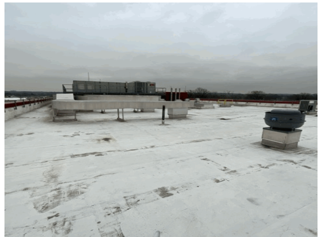
Roof 1 - South View
