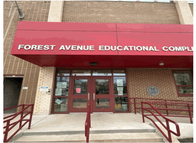
Facade A - Forest Avenue
