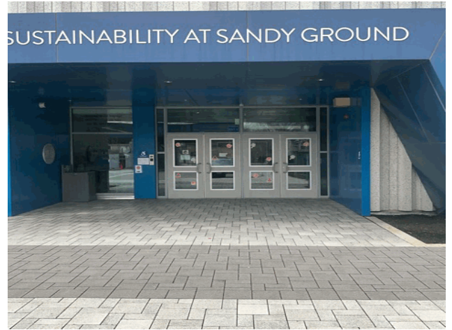
Facade A - Bloomingdale's Road
