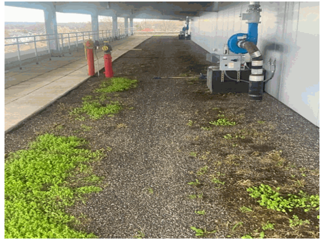
Roof 1 - East View
