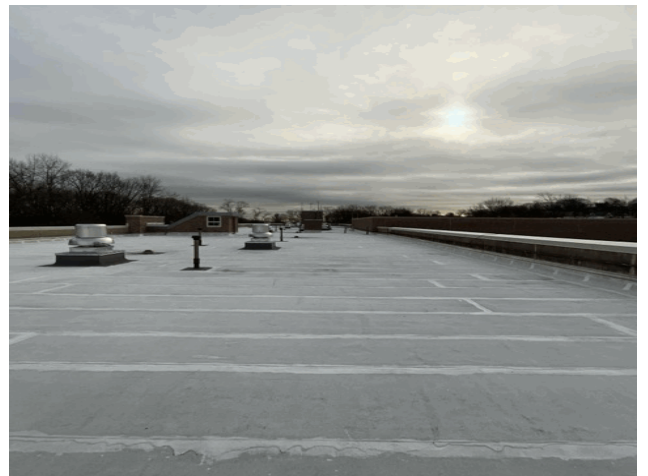
Roof 1 - East View
