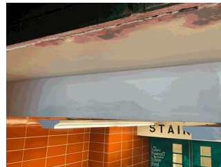
Stair A/2 shown, also Stairs A/3, C/2, D/3, Room 213 and Gymnasium
