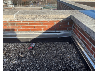
Roof 1 at Facade O
