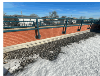
Facade A on Roof 1
