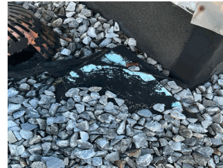
Roof 1 at Bulkhead BH1
