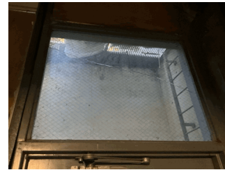
Areaway AW1 Boiler Room Exit Door
