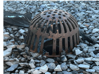
Roof 1 at Bulkhead Bulkhead BH1
