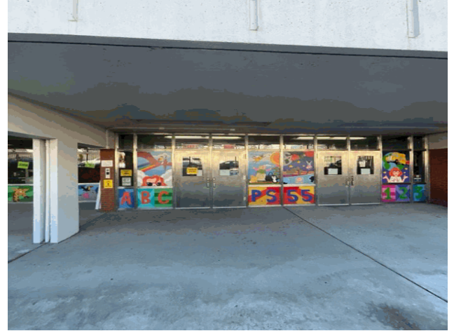
Facade A - Osborne Street
