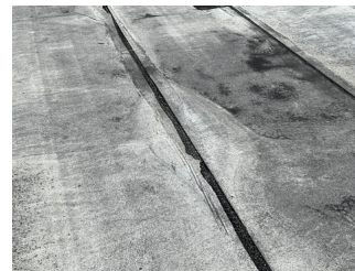
Roof 1 at Bulkhead BH3
