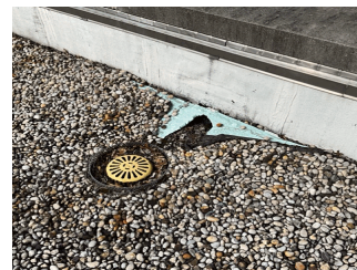
Facade H at Roof 2
