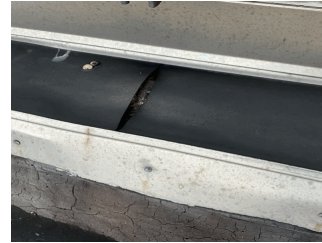
Facade E at Roof 3
