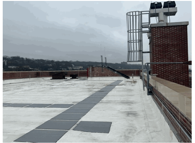
Roof 1 - North View
