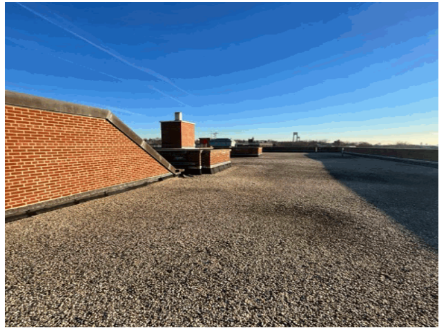
Roof 1 - Northeast View
