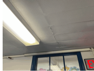
Corridor near Room 317
