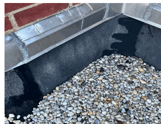
Facade A at Roof 1
