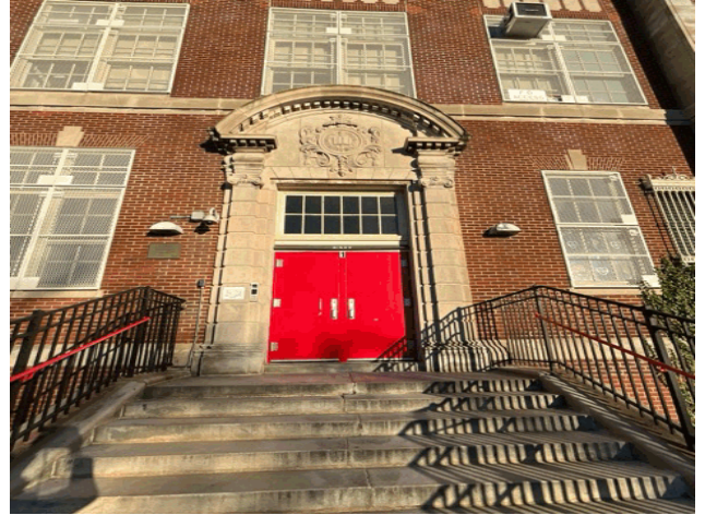
Facade A - Reid Avenue
