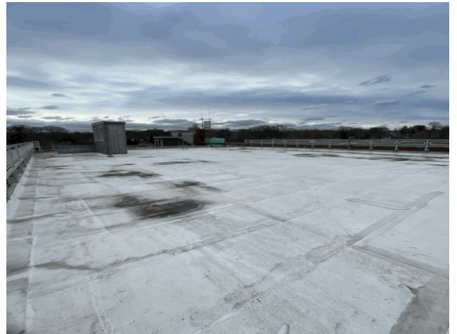
Roof 1 - East View
