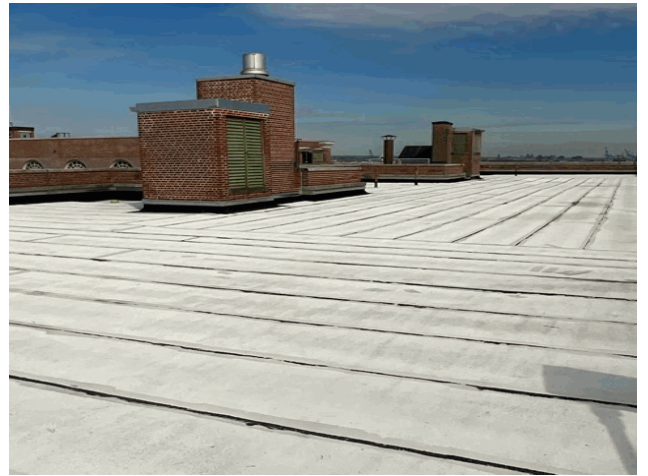
Roof 1 - Northwest View
