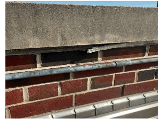
Roof 1 - Facade F
