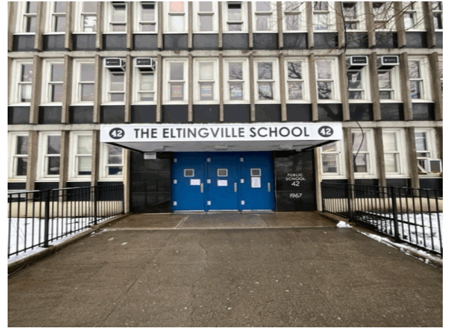
Facade A - Genesee Avenue
