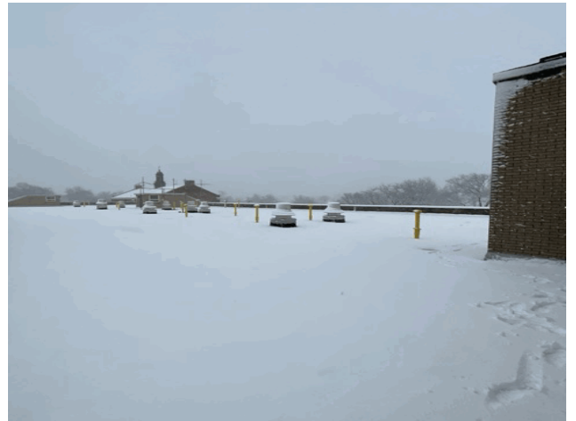
Roof 1 - East View
