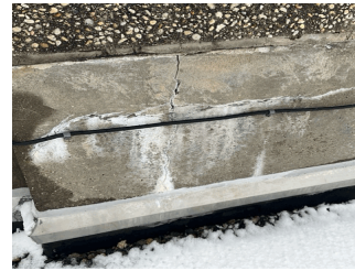
Facade B at Roof 1
