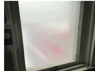
Room 325 (cloudy glazing)
