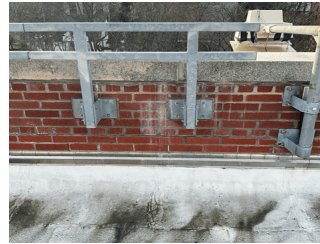
Facade A on Roof 1
