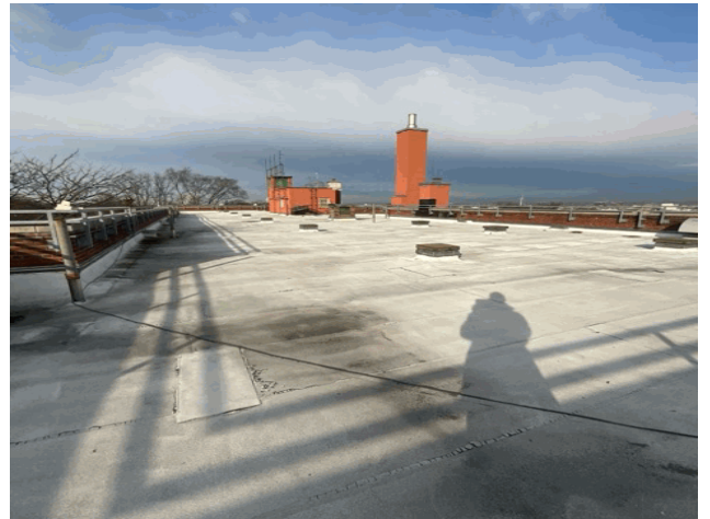
Roof 1 - West View
