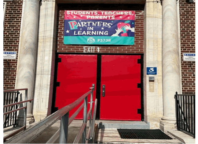
Facade A - Henderson Avenue
