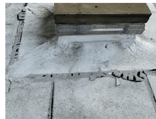
Roof 1 near Facade B
