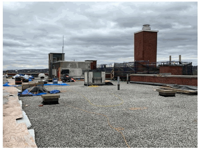
Roof 1 - North View
