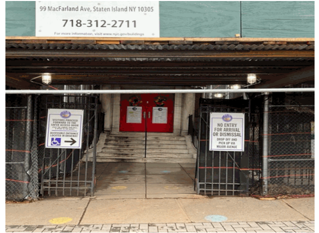
Facade A - McFarland Avenue
