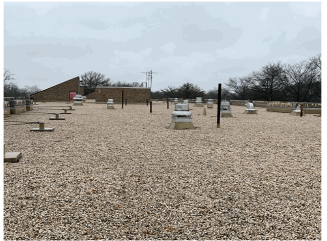
Roof 1 - North View
