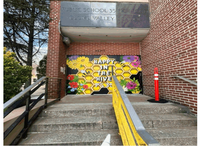
Facade A - Foote Avenue
