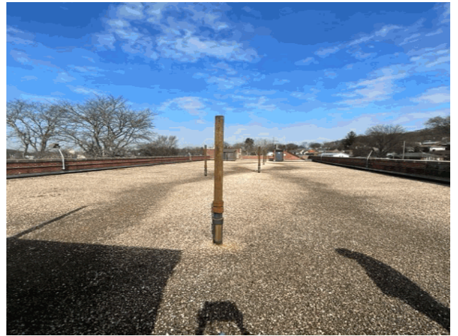
Roof 1 - North View
