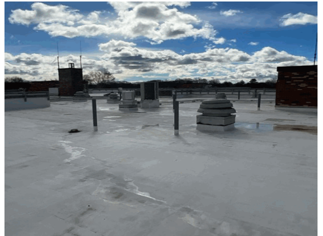
Roof 1 - East View
