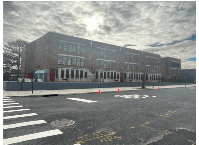
Corner of Barlow Avenue and Elverton Avenue - East View
