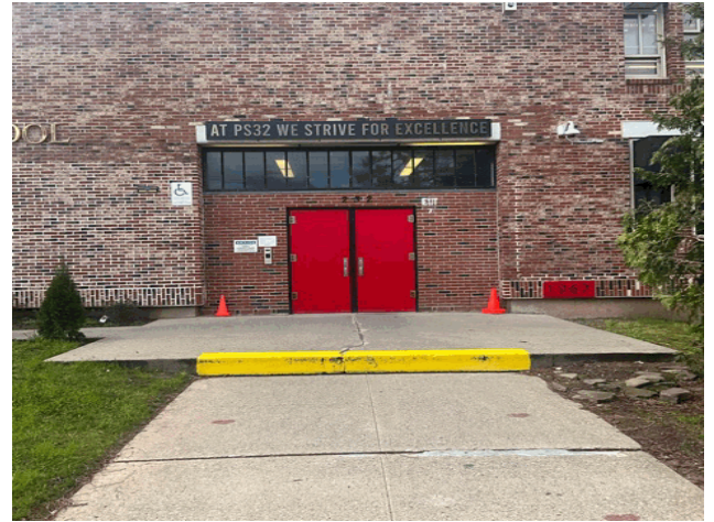
Facade A - Barlow Avenue
