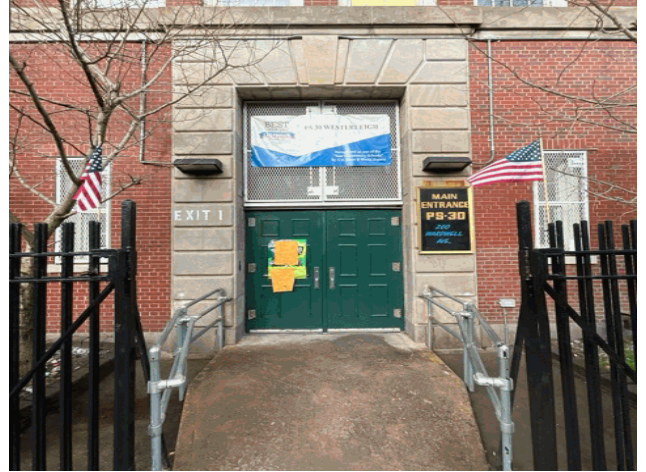
Facade A - Wardwell Avenue
