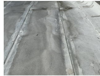
Roof 1 near Bulkhead BH2
