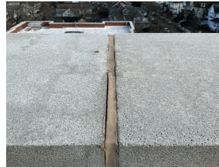
Facade A on Roof 1
