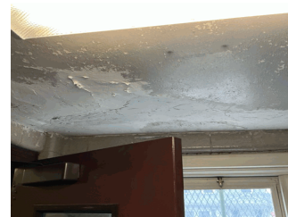
Exit 7 Vestibule (Stair F at Basement)
