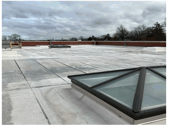
Roof 3 - North View
