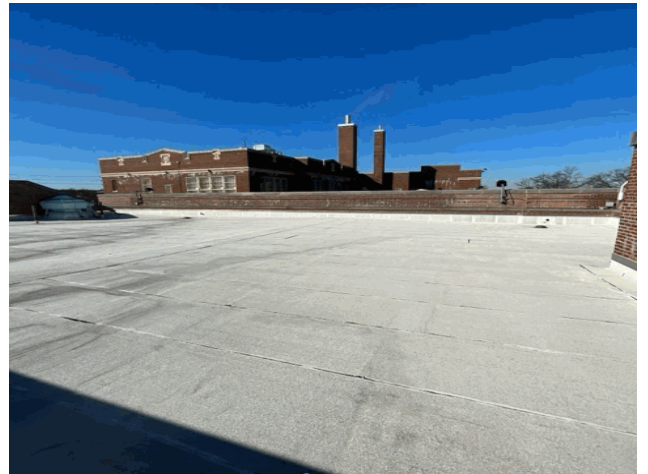
Roof 5 - South View
