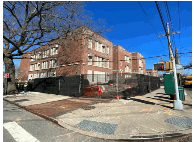
Corner of Victory Boulevard and Slossen Avenue - North View
