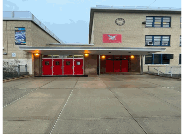
Facade A - Natick Street
