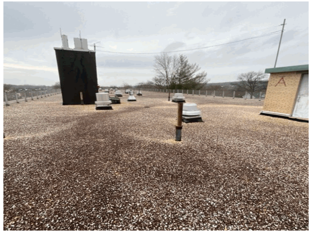
Roof 1 - West View
