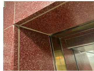
Corridor near Stair A/1 shown, also in Gymnasium
