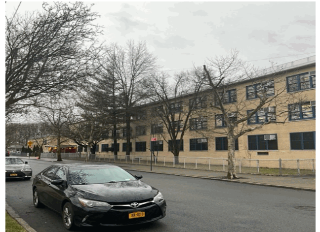
Corner of Natick Street and Maplewood Avenue - South View
