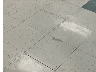
Corridor near Room A105
