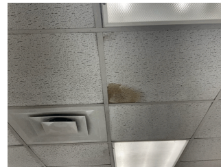
Room A203 shown, also Room A224 and 2nd Floor Corridor
