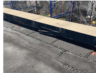
Roof 5 - Facade G
