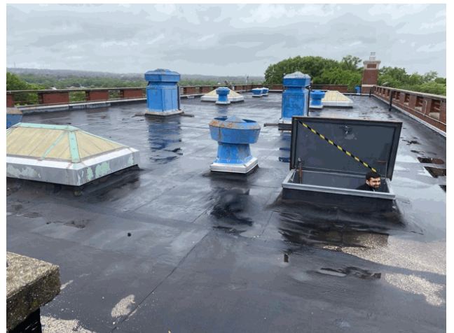
Roof 1 - South View
