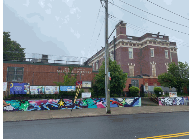
Walker Place - North View
