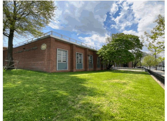
Corner of Broadway and Henderson Avenue - Southeast View
