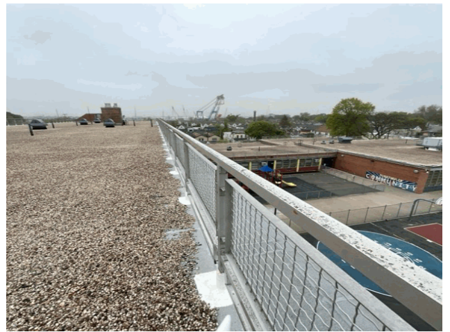
Roof 1 - North View
