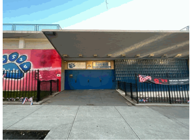
Facade A - Daniel Low Terrace
