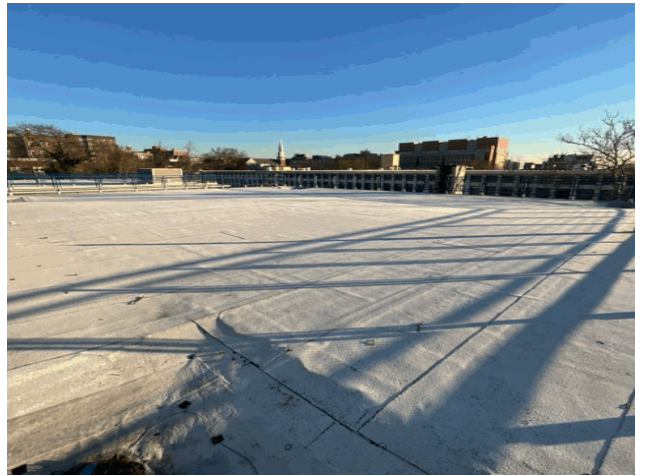
Roof 2 - North View
