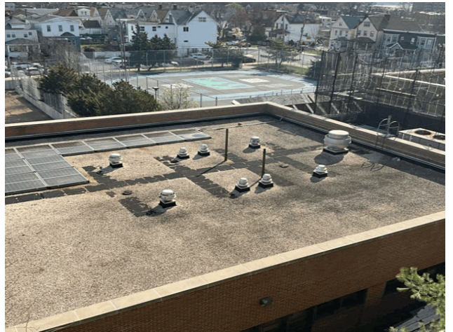
Roof 3 - East View
