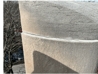
Facade A on Roof 6
