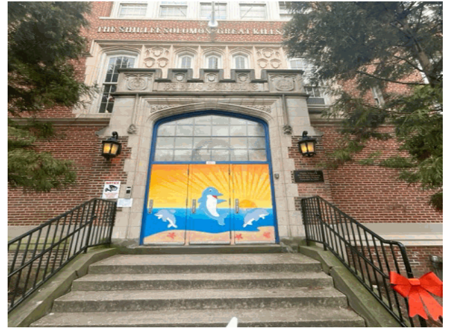
Facade A - Lindenwood Road
