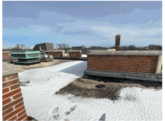
Roof 1 - East View
