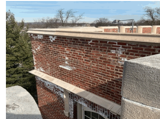
Facade A on Roof 1
