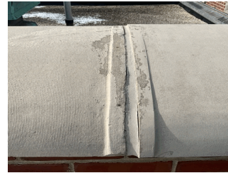
Facade A on Roof 1
