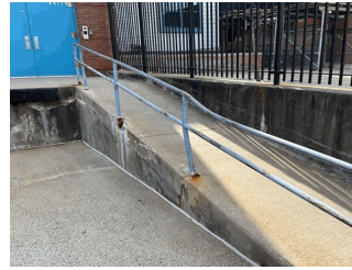
Loading Dock Ramp
