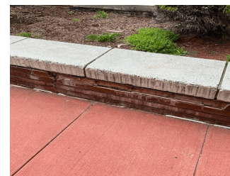
Main Entrance Ramp
