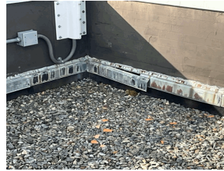
Facade A on Roof 1
