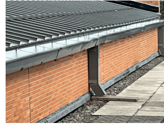
Facade I on Roof 2
