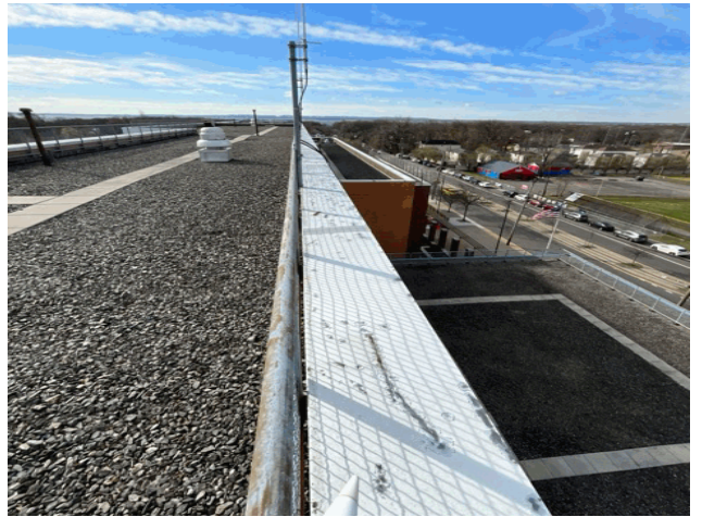
Roof 4 - South View
