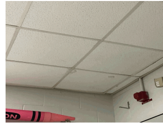
Room 258 (custodian's office)
