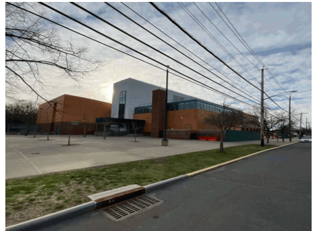
Corner of Page Avenue and Academy Avenue - East View
