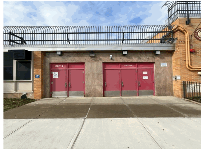
Facade A - South Goff Avenue
