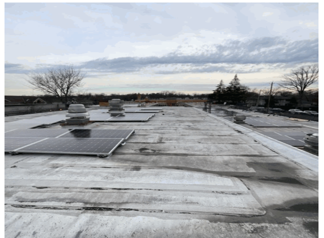
Roof 2 - North View
