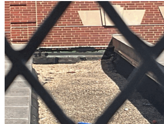
Roof 3 at Facade C
