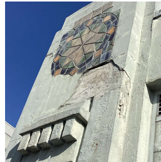
Facade D - Roof 2
