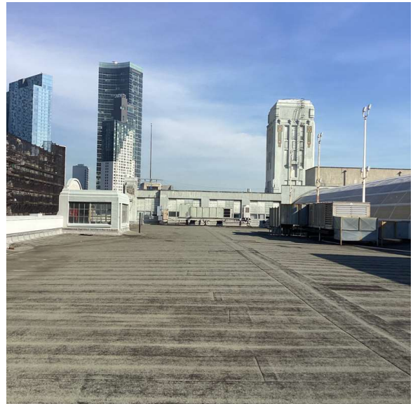
Roof 1 - North View
